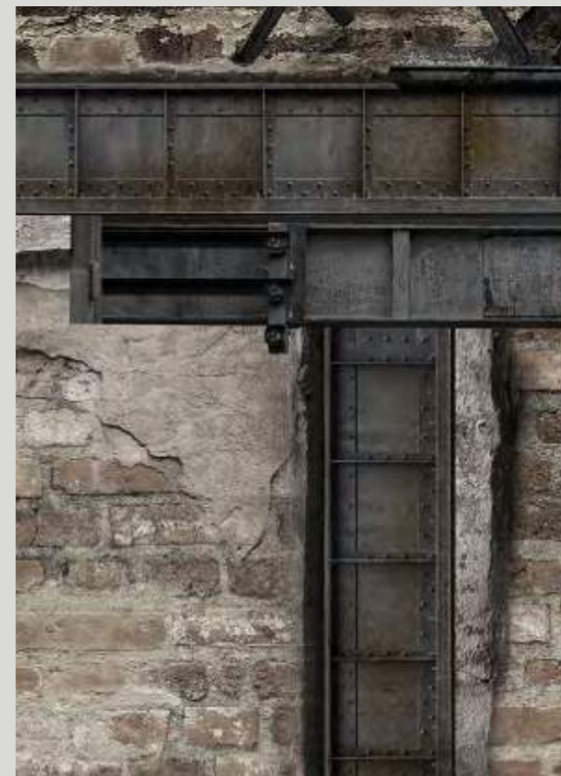
Brick WP08078 Parete in mattoni con putrella. Brick wall with beam.
